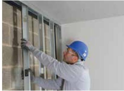
Gypframe 'I' Studs are friction-fitted vertically at the required centres within the channel sections to form the framework. Additional framing is installed as required to support heavy fixtures.
