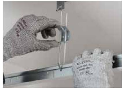
Use CasoLine QUICK-LOCK GRID Hangers to suspend the CasoLine QUICK-LOCK GRID 24/38 Main Tee.
