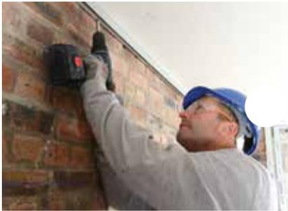
Gypframe GL8 Track is fixed to perimeters at 600mm centres with the longer leg towards the lining, using appropriate fixings.
