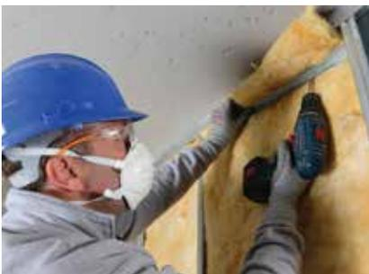
Isover Acoustic Roll is added to the partition cavity.
