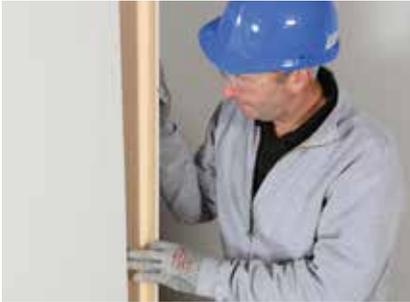
At reveals and external angles the lining is run past the corner and the insulating backing is cut back so as to form a neat junction with the reveal board or wall lining.
