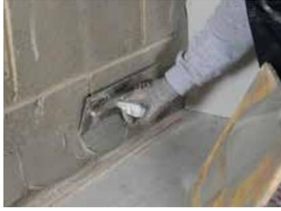
A continuous fillet / ribbon of Gyproc Plasterboard Compound is applied to the wall perimeter and around all services and openings as board fixing proceeds. This is particularly important if the lining is designed to act as an air barrier to achieve building airtightness.
