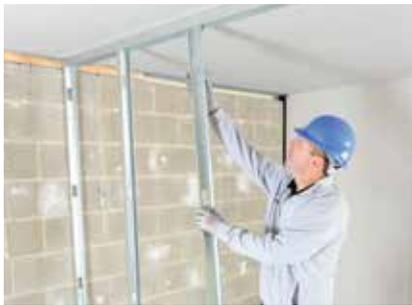
Gypframe studs are then friction fitted into the Gypframe Deep Flange Floor & Ceiling Channels at required centres.
