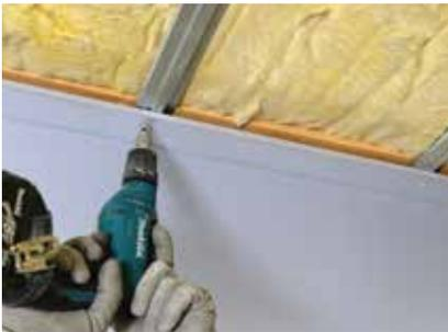
When fixing boards, care must be taken to ensure that the plasterboard fixing screws do not make contact with the joists.
