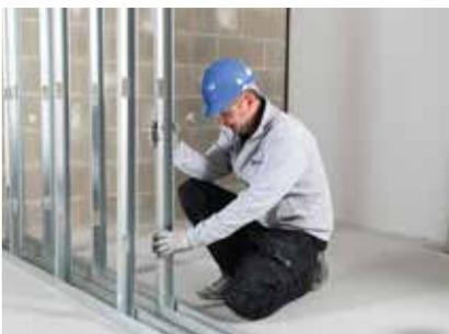
Gyproframe 'C' Studs are then friction fitted into the Gyproframe Floor & Ceiling Channels at the required centres. Door openings are constructed to the Heavy and Severe Duty Rating door detail.
