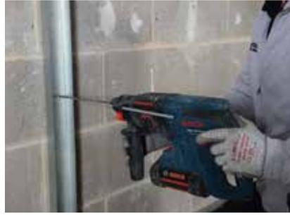
Gyproframe Starter Channels are suitably fixed to vertical abutments. The perimeter of the partition is sealed with Gyproc Sealant.
