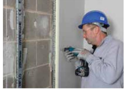
A continuous fillet / ribbon of Gyproc Plasterboard Compound is applied to the wall perimeter and around all services and openings as board fixing proceeds. This is particularly important if the lining is designed to act as an air barrier to achieve building airtightness. Boards are screw-fixed to all Gypframe MF10 Channel supports. Screw lengths should be selected to avoid contact with the masonry background.
