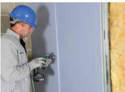
When applying multiple layers of board, ensure that all board joints are staggered on both sides of the partition.
