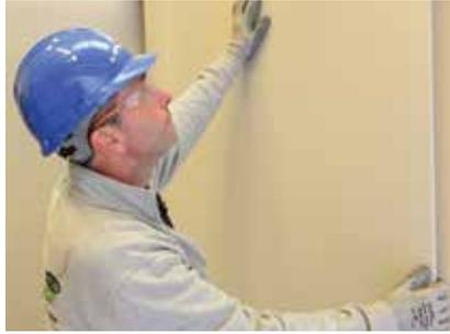
Boards are 'tapped' into position, lifted tight to the ceiling using a footlifter and supported until the adhesive sets. Further boards are installed, lightly butted together, to complete the lining.
