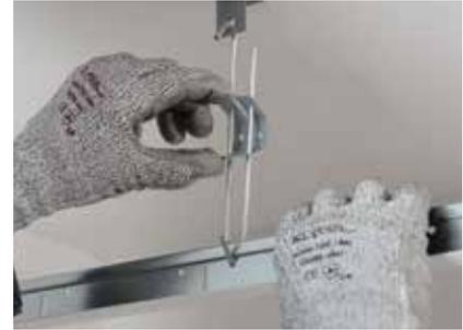
Use CasoLine QUICK-LOCK GRID Hangers to suspend the CasoLine QUICK-LOCK GRID 15/38 Main Tee.
