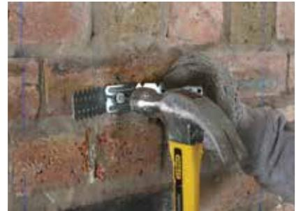
Vertical lines are marked on the wall at 600mm intervals to indicate Gypframe GL2 or GL9 Bracket fixing centres. Horizontal lines are marked at 800mm centres to determine individual bracket positions. Gypframe Brackets are then fixed into position.
