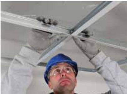
Install 600mm and/or 1200mm CasoLine QUICK-LOCK GRID 15/38 Cross Tee as required.
