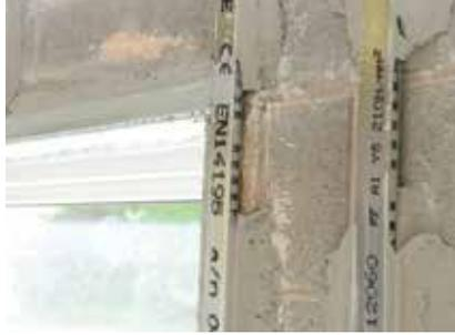
At angles and reveals, Gypframe MF10 Channels are installed close to the corner to provide support. Door and window openings are framed with Gypframe MF10 Channels. At window openings, the channel at the head forms a ground for fixing curtain track. Where a partition abuts, an additional Gypframe MF10 Channel is installed to provide a fixing ground. Board fixing can proceed once the adhesive has fully set.
