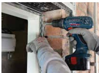
Gyproc Edge Bead can be fixed to window or door frames to provide edge protection to the reveal and soffit linings.
