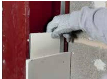
Additional layers of Glasroc F FIRECASE are fixed as before, with staggered joints. For single layer steel beam encasements, additional strips of Glasroc F FIRECASE are installed behind the ends of the facia board-ends so as to seal the joints.
