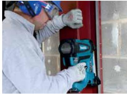
For two or three-sided protection to steel beams or columns, Gypframe FEA1 Steel Angles are located to both sides of the wall / soffit flange and secured using appropriate fixings.
