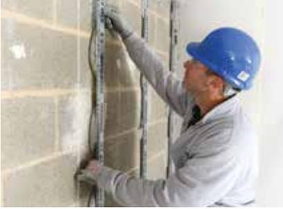
The board edge and centre positions are marked on the wall and dabs of Gyproc Plasterboard Compound are applied progressively to the wall to each vertical line.
