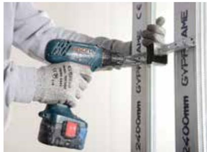
The Gypframe 92 S 10 'C' Studs are then braced together in pairs with either staggered Gyproc GAB3 Acoustic Braces,
