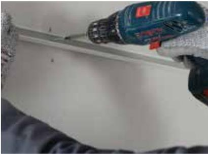
Measure and mark the required ceiling height, then fix the CasoLine QUICK-LOCK GRID WA02 Wall Angle or WA03 Wall Angle around the perimeter of the ceiling area to suit.
