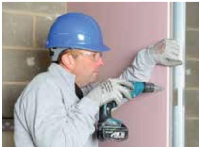
The appropriate lining boards are screw-fixed to framing members to form the lining, except 6mm Glasroc F MULTIBOARD, which is screw-fixed to the Glasroc F FIRECASE linings.
