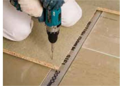
Flooring is laid across the Gypframe SIF Floor Channels and screw-fixed through the Gyproc Plank to the channel flange on one side only, using Gypframe SIF5 Floor Screws. It is important to ensure that no fixings are allowed to connect the Gypframe SIF Floor Channels to the joists.
