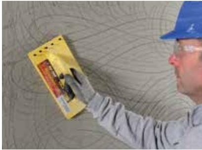
The final coat is ruled to an even surface and lightly scratched to form a key for Gyproc Finish Plasters.
