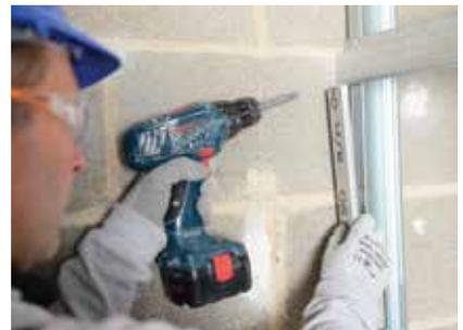
Gypframe RB1 Resilient Bars are installed vertically to abutment and door studs to accept perimeter fixings for the Gyproc plasterboard linings.
