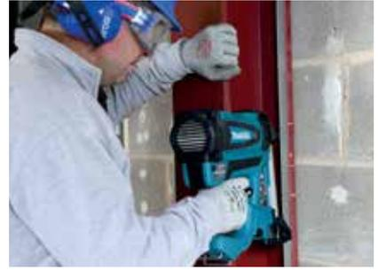
For two or three-sided beams or columns Gypframe GA2 Steel Angle is located to both sides of the wall / soffit flange and secured using appropriate fixings.
