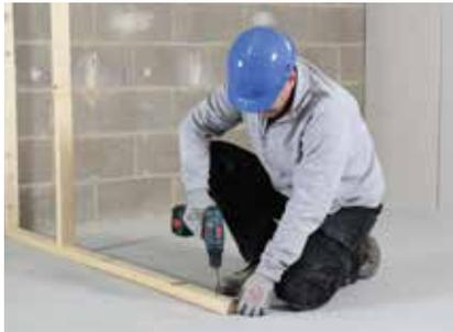
Timber framing is fixed to the perimeter, abutments, and to frame any openings, using suitable fixings. Timber studs are fixed at specified centres.
