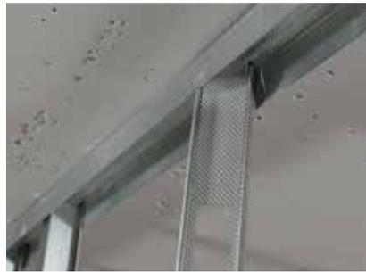
The studs are then friction fitted into the Gypframe Channels, alternating the direction of the clip to create a staggered stud framework.
