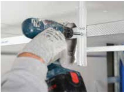
Gypframe MF7 Primary Support Channels are fixed to the hangers with Gyproc Wafer Head Jack-Point Screws, two per hanger.
