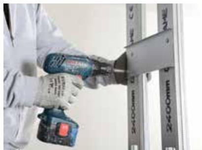
The two frameworks are braced with Gyproframe 99 FC 50 Fixing Channel attached to the Gyproframe 'C' Studs with Gyproc Wafer Head Drywall Screws, two screws per junction.
