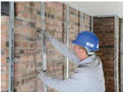
Gypframe GL1 Lining Channels are friction-fitted into the track, extending if required.
