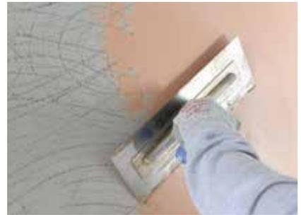
Once the Gyproc undercoat plaster has set, Gyproc Finish Plaster is applied with firm pressure, built out to the required thickness in two applications and trowelled to a smooth matt finish. In some circumstances it may be necessary to control the suction with Gyproc GypPrime. Good site practice should be followed, as outlined in *BS EN 13914 - 2 Design considerations and essential principles for internal plastering*.
