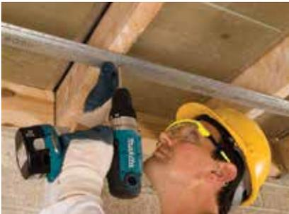
Gypframe RB1 Resilient Bars are installed to the underside of the joists with Gyproc Drywall Screws.
