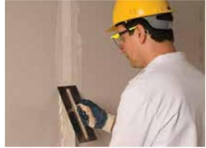
Where there is an increased risk of cracking, or where joints exceed 3mm, the joints are reinforced with Gyproc Paper Joint Tape bedded in Gyproc plaster.
