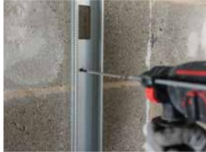
Gypframe 92 S 10 'C' Studs are fixed at abutments and door openings in two rows.
