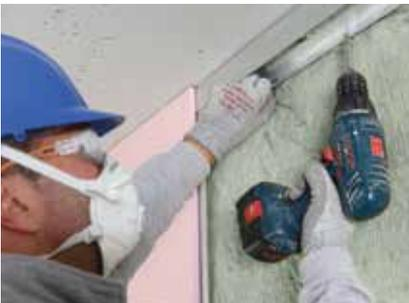
Stone mineral wool insulation (by others) may also be added to the partition cavity for increased performance.
