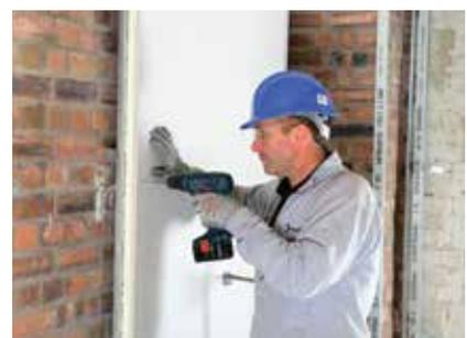
Gyproc plasterboards or thermal laminates are then fixed to all framing members with Gyproc Drywall Screws.
