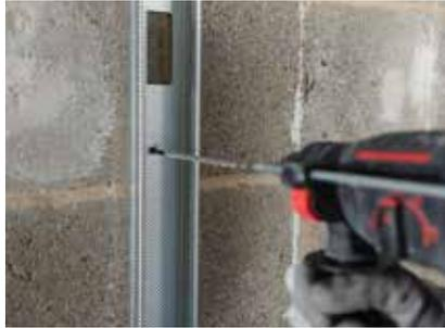
Gypframe Studs are suitably fixed to abutments.
