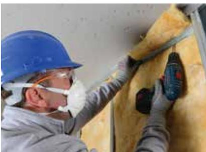
Isover Acoustic Roll insulation is added to the partition cavity for optimal acoustic performance.
