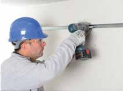
Gypframe GL8 Track is fixed at the perimeter of the room with the longer leg at the bottom.
