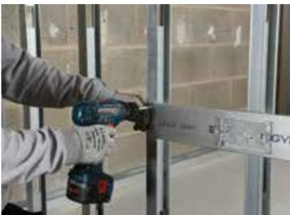
M&E services can be located within the partition cavity. Care should be taken to prevent bridging, for example socket boxes making contact with the opposing studs.
