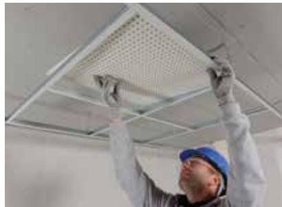
CasoLine QUICK-LOCK GRID is self-squaring, so with the CasoLine QUICK-LOCK GRID 15/38 Cross Tee in place to form the grid, tiles can be easily laid into place.
