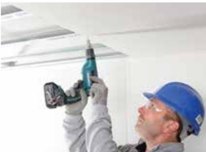
Gyproc plasterboards, Glasroc specialist boards, Gyptone boards or Rigitone boards are then screw fixed to the Gypframe MF5 Ceiling Sections and Gypframe MF6 Perimeter Channels with Gyproc Drywall Screws.
