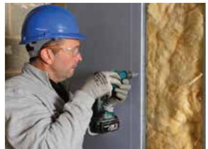
Gyproc SoundBloc plasterboards are then screw fixed to alternate Gypframe 'I' Studs and other framing members with Gyproc Jack-Point Screws.
