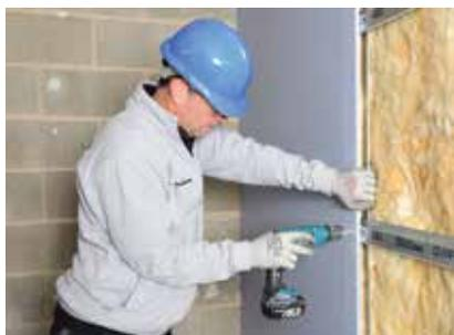
Gyproc plasterboards are fixed with Gyproc Drywall Screws to the Gypframe RB1 Resilient Bars with all joints staggered. Where Gyproc Plank is required as an inner layer, it is fixed horizontally to the Gypframe RB1 Resilient Bars at each bar position.
