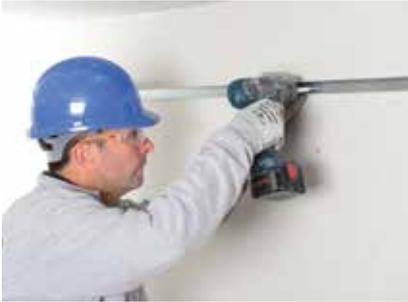
Gypframe MF6 Perimeter Channels are fixed to the perimeter walls at 600mm centres.
