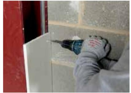
Glasroc F FIRECASE boards are cut to width and fixed to the Gypframe FEA1 Steel Angles with Glasroc F FIRECASE Screws.
