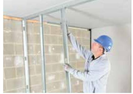
Gypframe 'I' Studs or 'C' Studs are then friction fitted into the Gypframe Channels at required centres.
