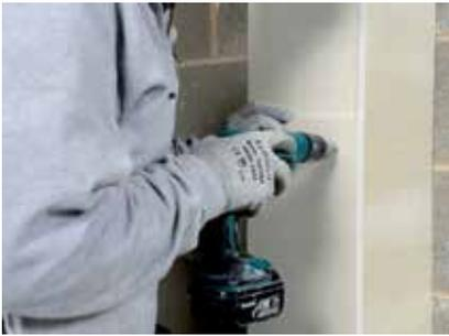
For four-sided protection to steel columns, Glasroc F FIRECASE boards are positioned and fixed board to board using Glasroc F FIRECASE Screws.
