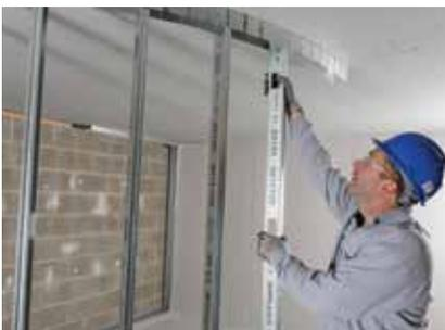
Gypframe studs are fitted and fixed into the Gyproc 72 EDCL 80 Curvelyner Channels at the required centres. If a deflection head is required, the studs should not be fixed into the head channel and alternative temporary support may be required to stabilise the stud at the head whilst boarding proceeds.
