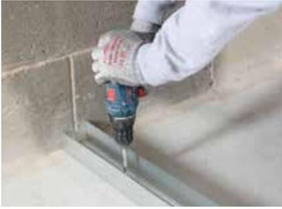
The appropriate Gyproframe channels, are suitably fixed to the floor and soffit of the structure. Gyproc FireStrip is used on the channel at the soffit.
