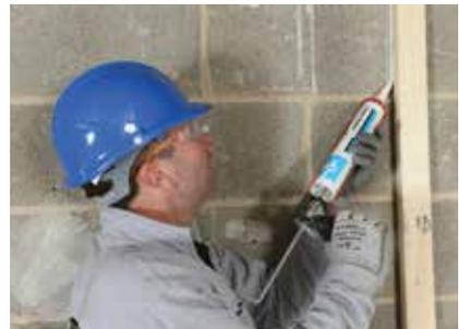
The perimeter of the partition is sealed on both sides with Gyproc Sealant.
