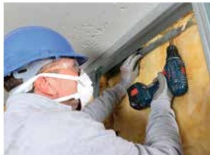
Insulation is added to the partition cavity.
