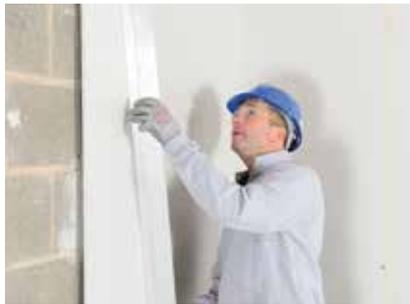
Further boards are installed, lightly butted together, to complete the lining.
