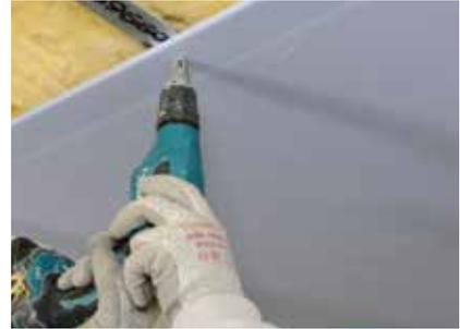
Gyproc plasterboards are fixed to the underside of Gypframe RB1 Resilient Bars with Gyproc Drywall Screws.
