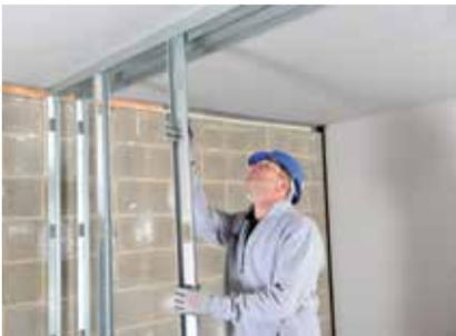
Gypframe 92 S 10 'C' Studs are then friction fitted into the Gypframe Channels at the required centres, and door openings are constructed to the Heavy and Severe Duty Rating door detail.
