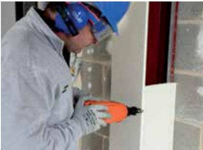
Where Glasroc F FIRECASE boards abut they can be fixed together with either Glasroc F FIRECASE Screws or Glasroc Staples.
