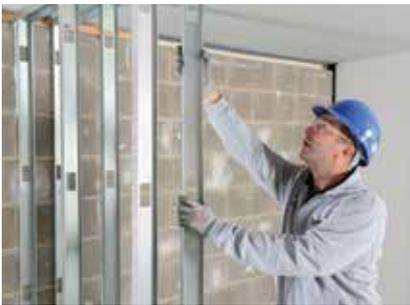
Gypframe 'I' Studs are then friction fitted into the Gypframe Channels at the required centres.
