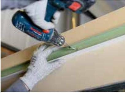
CasoLine quick-lock GRID Shadowline Moulding CLSM04 is fixed to the wall at 300mm centres.
