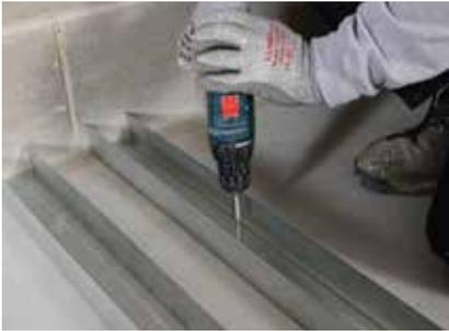
Gyproframe Floor & Ceiling Channels are suitably fixed to the floor and soffit in two rows.
