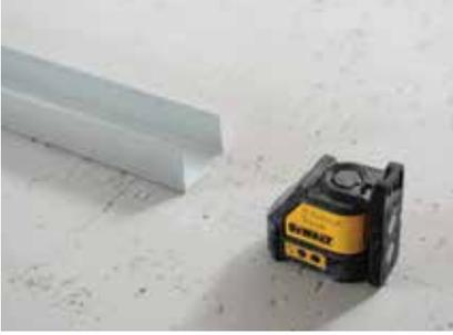
Gypframe Floor & Ceiling Channels are suitably fixed to the floor and soffit.
