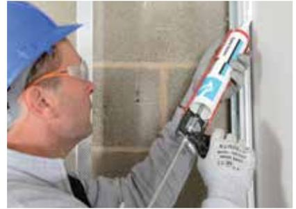
The perimeter of each frame is then sealed with Gyproc Sealant.
