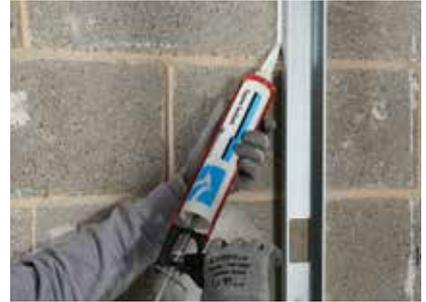
The perimeter of the partition is then sealed with Gyproc Sealant except where Gypframe RB1 Resilient Bars are to be installed on that side. Where Gypframe RB1 Resilient Bars are to be installed, the Gyproc Sealant is applied to the perimeter of the first layer of board.
