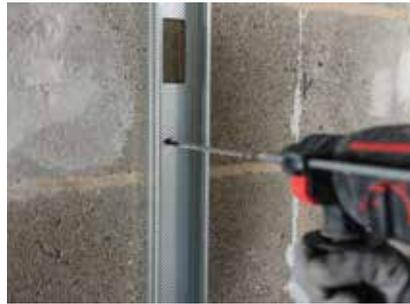
Gypframe 'C' Studs are suitably fixed at abutments and door openings.
