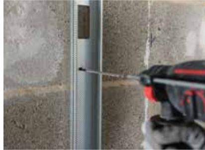
Gypframe Studs are suitably fixed to abutments.
