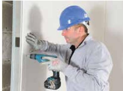
Boards are screw-fixed to framing members to form the lining. Horizontal board joints should be backed with Gypframe GFS1 Fixing Strap or Gypframe GFT1 Fixing 'T'.
