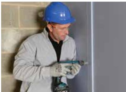
Gyproc plasterboards are screw-fixed to all timber supports with Gyproc Drywall Screws, or to the Gypframe RB1 Resilient Bars with Gyproc Drywall Screws.
