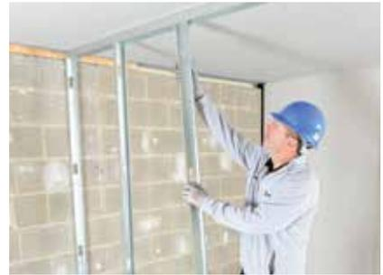
Gypframe studs are then friction fitted into the Gypframe Floor & Ceiling Channels at required centres.
