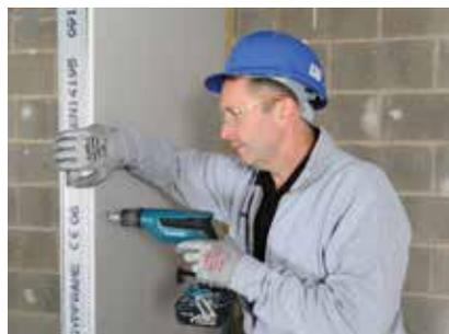
Gyproc plasterboards or Glasroc specialist boards are fixed to the Gypframe framework with Gyproc Drywall Screws.
