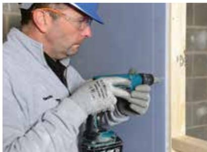
Horizontal board joints are backed with timber noggings or Gypframe RB1 Resilient Bars as required.
