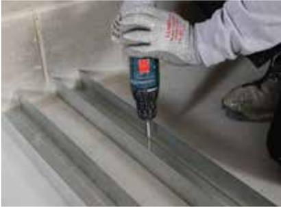
Gypframe Floor & Ceiling Channels are suitably fixed to the floor and soffit in two rows.
