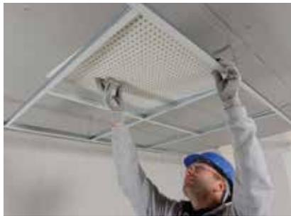
CasoLine QUICK-LOCK GRID is self-squaring, so with the CasoLine QUICK-LOCK GRID 24/38 Cross Tee in place to form the grid, tiles can be easily laid into place.
