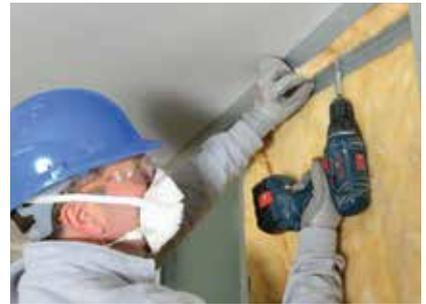
Isover Acoustic Roll can be added to the partition cavity for increased acoustic performance.
