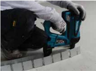
Gypframe 72 EDCL 80 Curvelyner Channels are suitably fixed to the floor and soffit, bent by hand to suit the required radius.
