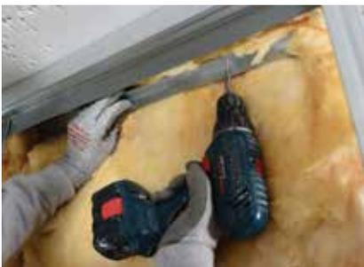
Isover insulation is added to the partition cavity for increased acoustic performance.
