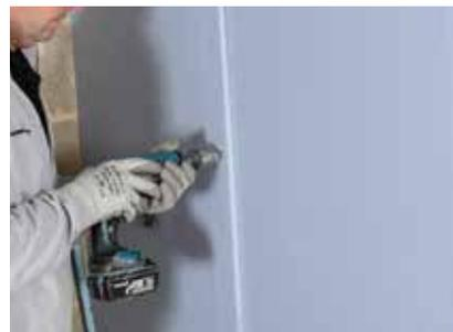
Gyproc plasterboards are then fixed to the Gyproframe framework with Gyproc Drywall Screws.
