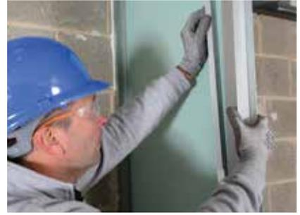
Gyproframe 'I' Studs or Gyproframe Tabbed 'I' Studs are friction fitted into the channels at 600mm required centres. Gyproc CoreBoard or 20mm Glasroc F FIRECASE is fitted between the studs on the shaft side, and held in place with appropriate Gyproframe Retaining Channels. Door openings are formed to the ShaftWall Access Door Details.
