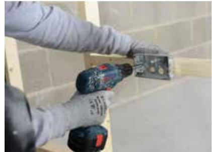
M&E services can be located within the partition cavity before the partition has been boarded. Timber noggings are fixed to support recessed switch boxes / socket outlets.
