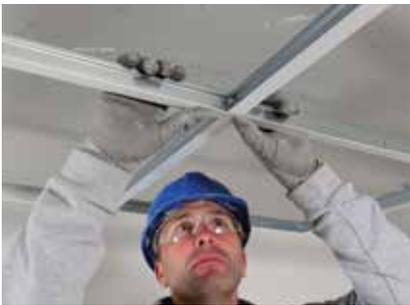
Install 600mm and/or 1200mm CasoLine QUICK-LOCK GRID 24/38 Cross Tee as required.
