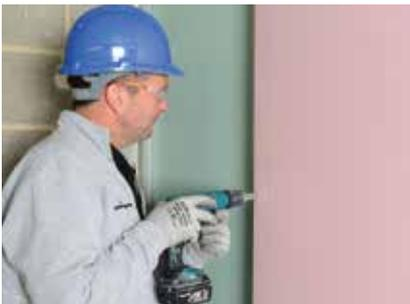
Gyproc plasterboard or Glasroc F FIRECASE are then fixed to the Gyproframe framework with Gyproc Drywall Screws or Gyproc Jack-Point Screws.
