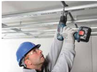
Gypframe MF5 Ceiling Sections are fixed to the underside of the Gypframe MF7 Primary Support Channels to form a grid with Gyproc Wafer Head Jack-Point Screws.
