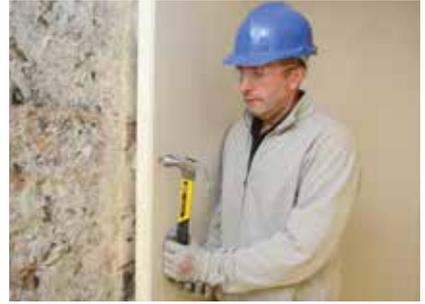
When installing Gyproc ThermaLine laminates in the DriLyner **RF** system, insert two Gyproc Nailable Plugs at mid height after Gyproc Sealant has set, as secondary mechanical fixings.
