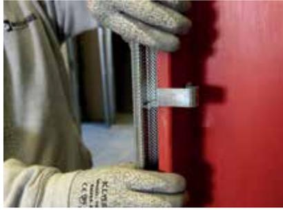
Gypframe GL1 Lining Channels are located over the clips to form the steel framework.
