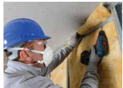
Isover Acoustic Roll insulation can also be included within the partition cavity for optimised acoustic performance.
