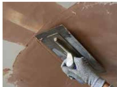
For best results Gyproc plaster is applied with firm pressure, built out to the required thickness in two applications and trowelled to a smooth matt finish. Good site practice should be followed, as outlined in *BS EN 13914 - 2: Design Considerations and Essential Principles for Internal Plastering*.
