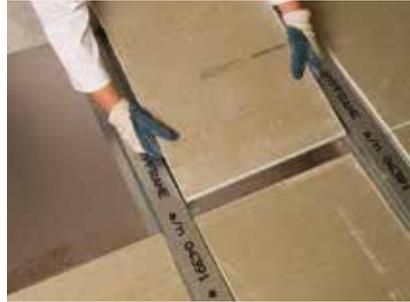
Gyproc Plank is cut neatly to fit between the channels.
