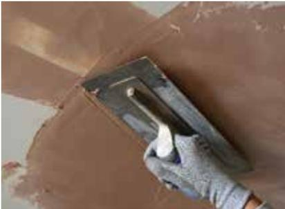
Gyproc plaster is applied with firm pressure, built out to the required thickness in two applications and trowelled to a smooth matt finish. Good site practice should be followed, as outlined in *BS EN13914 - 2: Design Considerations and Essential Principles for Internal Plastering*.
