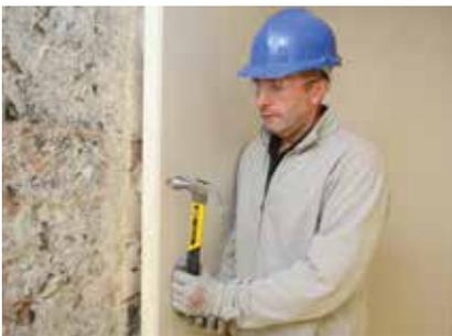
When installing Gyproc ThermalLine laminate in the **Drilyner π** system, insert two Gyproc Nailable Plugs at mid height after dabs have set, as secondary mechanical fixings.
