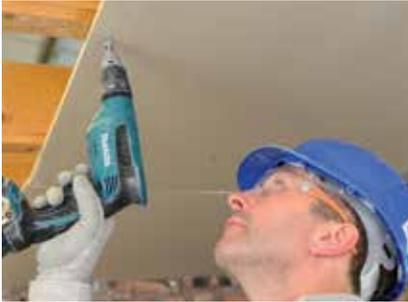
Gyproc plasterboards can be fixed directly to the underside of timber joists. Timber noggings are fitted, where required, between joists at room perimeters to support board edges. Noggings may also be required to support board edges in the field of the boards. Plasterboards are fixed to timber supports using Gyproc Drywall Screws.
