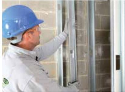
Gyproframe 'C' Studs are suitably fixed to abutments in two rows.
