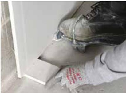
Lifted tight to the ceiling using a footlifter and supported until the adhesive sets.
