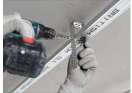
Gypframe GL1 Lining Channels are located into the perimeter track and each leg of the Gypframe GL2, GL9 or GL12 Brackets are screw-fixed to the Gypframe GL1 Lining Channels with Gyproc Wafer Head Drywall Screws.
