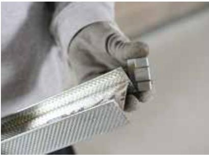
Gypframe SC1 or SC2 Spacer Clips are inserted to the top and bottom of the Gypframe 60 I 70 or 92 I 90 'I' Studs respectively.
