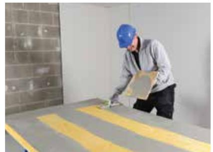
The fitting of Gypframe Skirting Plates over the bottom edge of the boards during installation provides a ground for subsequent skirting fixing.
