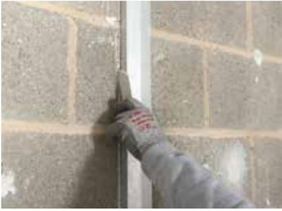
The board edge positions are marked on the wall, and Gyproc Plasterboard Compound is applied to the wall in dabs to support the boards.
