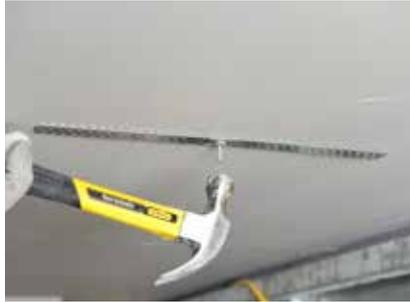
Gypframe GL2, GL9 or GL12 Brackets are fixed to the soffit at the required centres.
