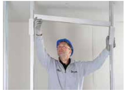
Door openings are constructed to the Heavy and Severe Duty rating door detail.
