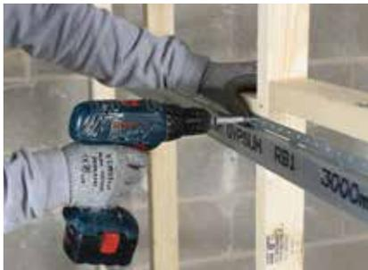
Where Gypframe RB1 Resilient Bars are required, these are fixed horizontally to the timber studs to one or both sides as specified.
