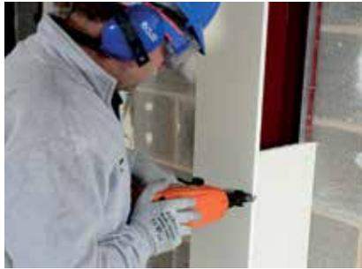
Board-end joints are backed using horizontal noggings formed from an appropriate Gypframe component: Gypframe GL1 Lining Channel, Gypframe GFS1 Fixing Strap or Gypframe GFT1 Fixing 'T'.
