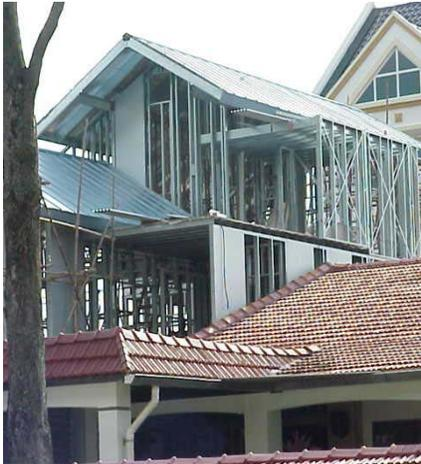
**Strong but Lightweight:** Steel has one of the highest strength-to-weight ratios of any construction material. This results in savings in the foundation required and the lightness also makes for easier on-site handling.
