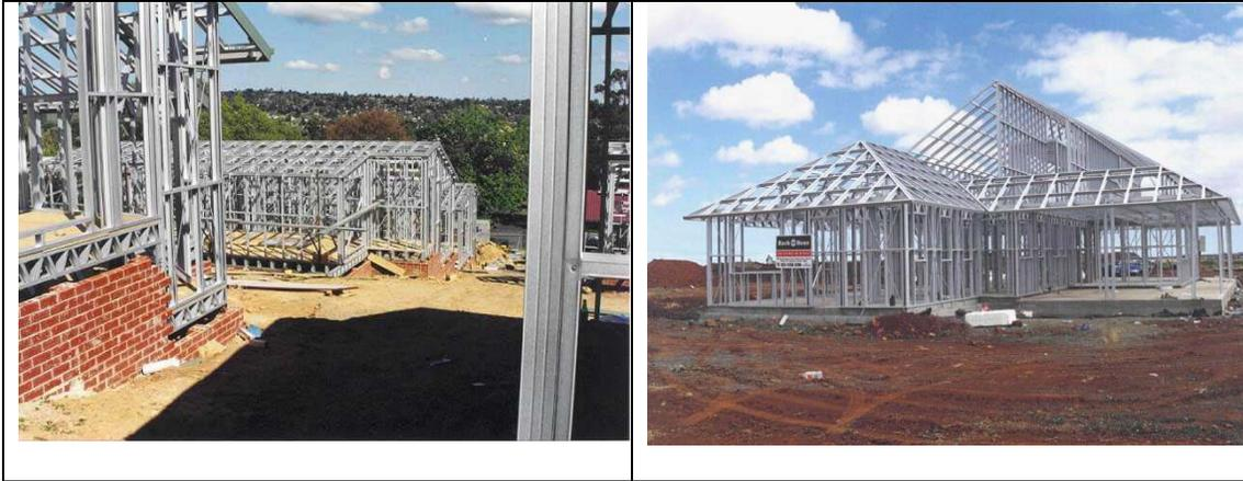
Figure 9.4 Load Bearing Wall Details & Installation
